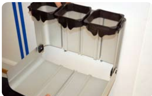
4 Place the GP15 on the two bottom screws
