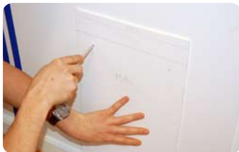
1 Place the template and make preholes/drilling guides
