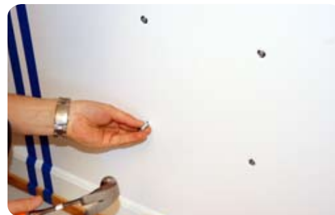
3 a) For plaster remove the two top screws and keep the two bottom ones with a 5mm gap to the wall
