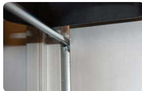
6 Use a long bit to tighten the two top screws
